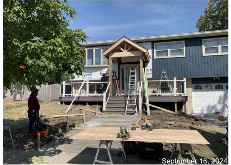
During construction (September 2024)
